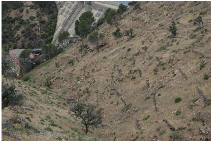
Figure 42. Contour-felled log debris barriers (Navas del Rey, Madrid). Photo: Sergio de Frutos
