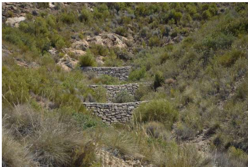
Figure 43. Dry masonry check-dam (Hellín, Albacete). Photo: Sergio de Frutos
