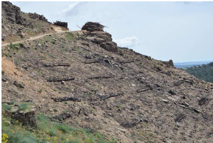
Figure 41. Mixed barriers made with burned logs and debris (Collado Mediano, Madrid). Photo: Sergio de Frutos
