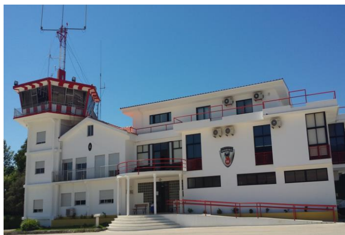
Figure 2. ENB Specialised Training Centre in Forest Fires. Source: ENB
