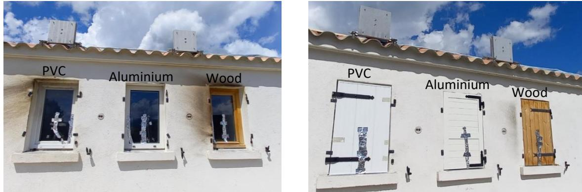
Figure 12: Photographs of the joinery a) Windows made of PVC (left), Aluminium (centre) and Wood (right) ; b) Shutters made of PVC (left), Aluminium (centre) and Wood (right)
